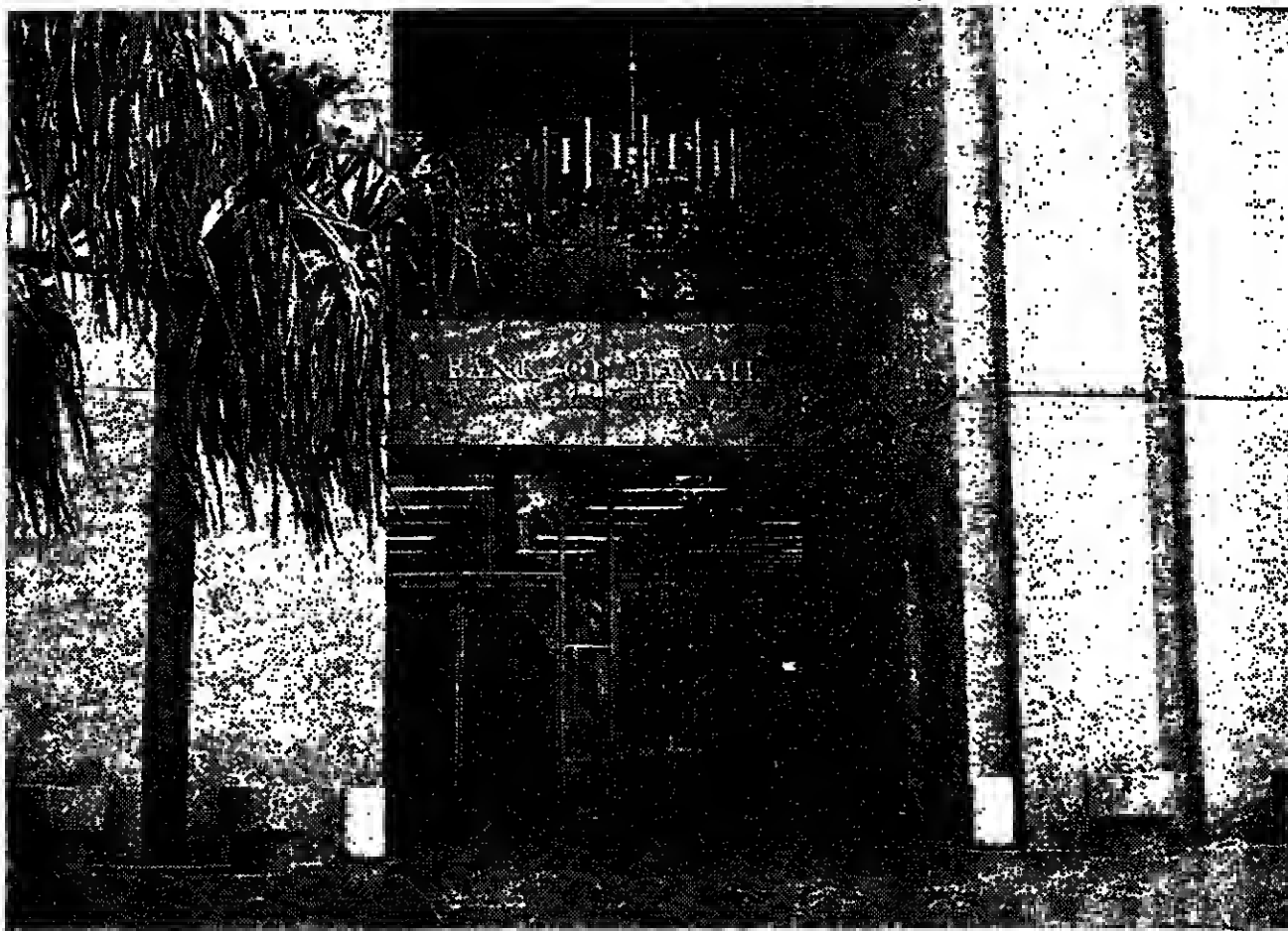
Bank of Hawaii Headquarters, Honolulu, Hawaii
